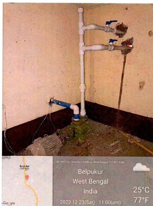
7.5 HP Pump to harvest Rainwater from reserve to overhead tank 2
