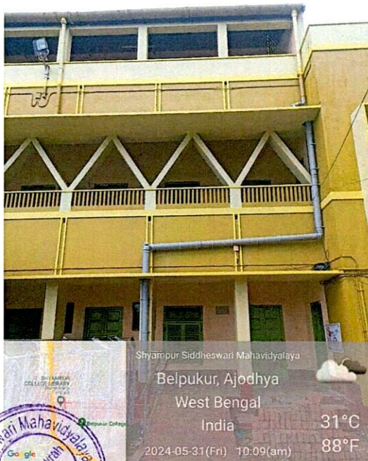
Rainwater collected through pipes destined to rainwater reserves
